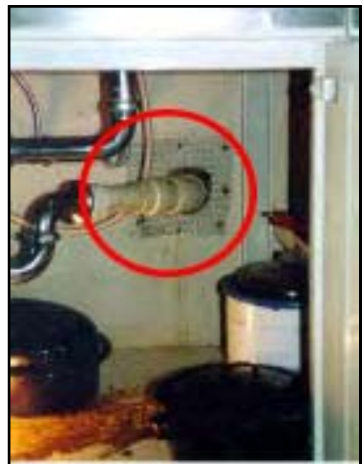
Use lath metal around pipes
